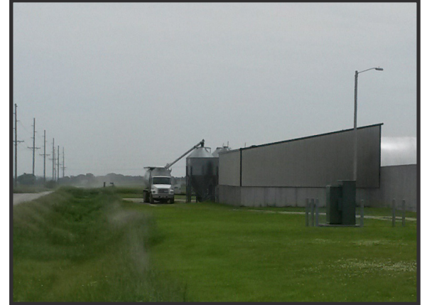
Drive and park in designated areas. Follow all posted signs.
